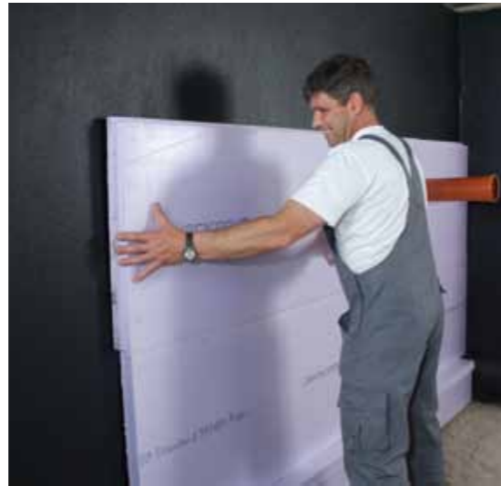
XPS boards completely bonded with KÖSTER Deuxan®
