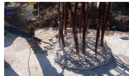
Removing protrusions, cleaning the pile head
