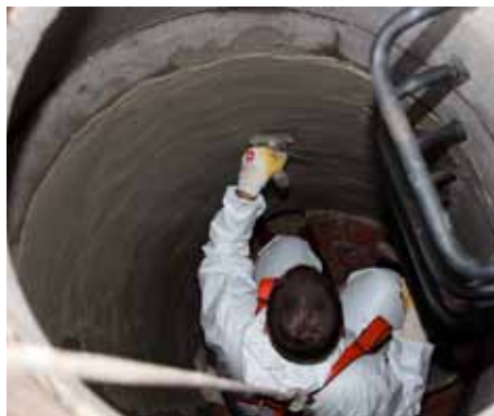
The mortar is applied to the moist substrate by trowel.
