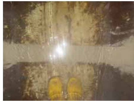
Very stable - even under flowing water
